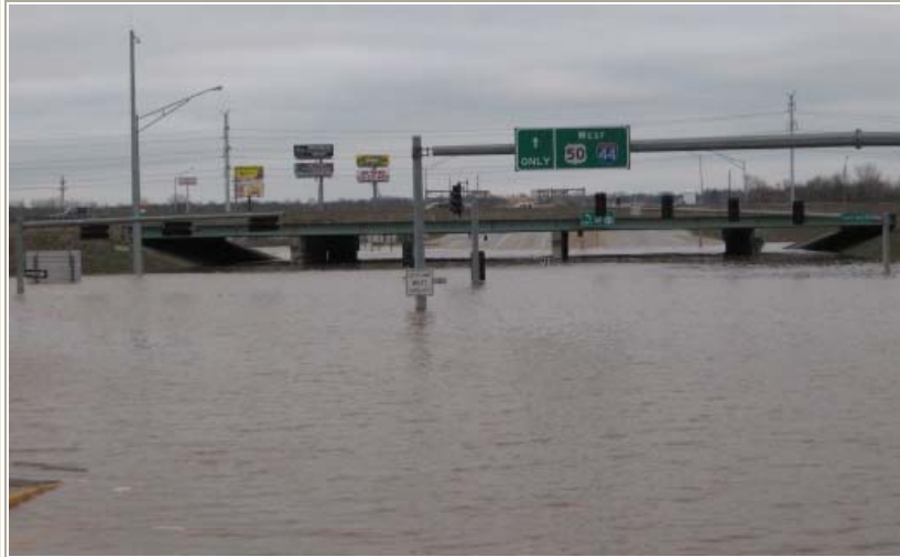
Figure 1: Flooding of Highway 141 at the Interstate 44 underpass
