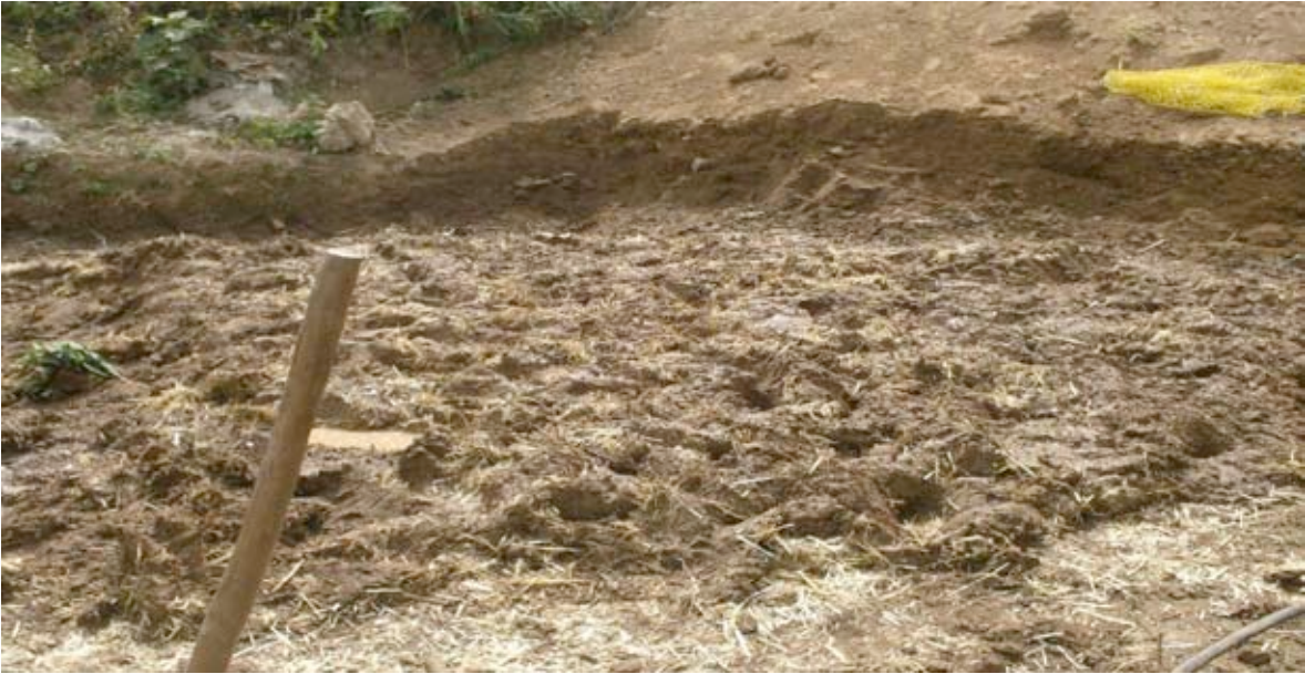
Photo No. 1. Clay commonly known as “barro”, mixed with straw and water.
