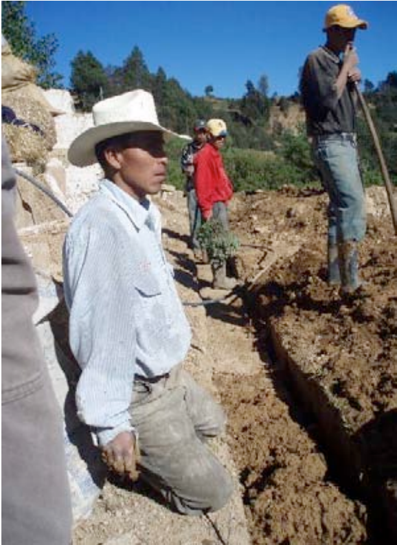
Photos No. 10 and 11: Placement of material to form the foundation.
