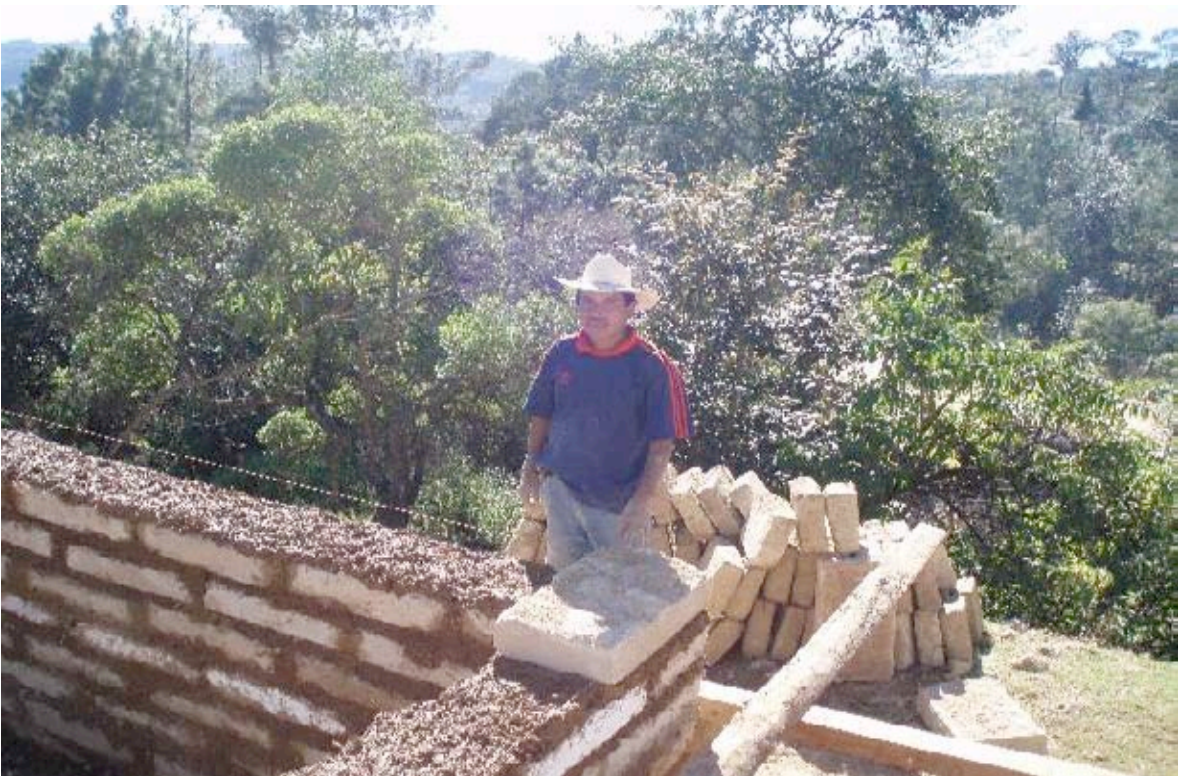
Photo No. 15: Placement of adobe mortar.
