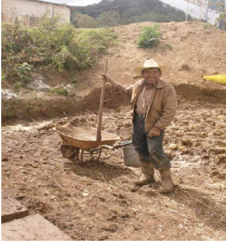
Photo No. 5: Preparation of the adobe mixture.
