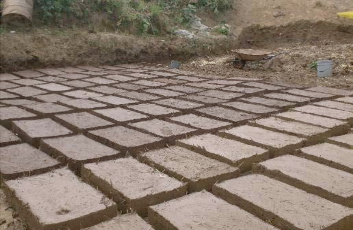
Photo No. 8: Adobes after wooden frames have been removed.
