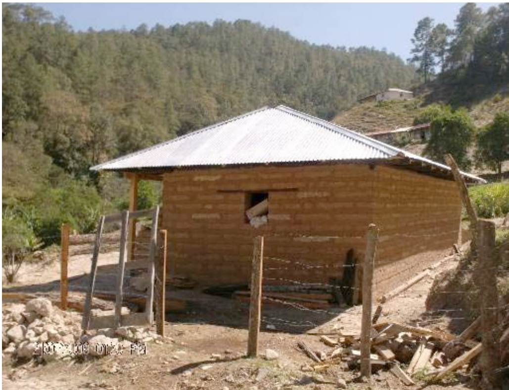
Photo No. 17: Board placed above window to support the overlying adobe.
