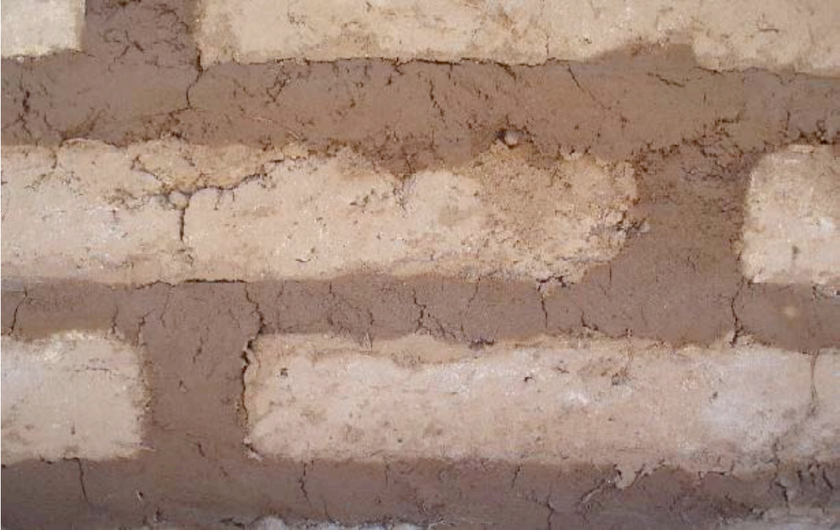
Photo No. 14: Placement of overlapping adobe bricks.
