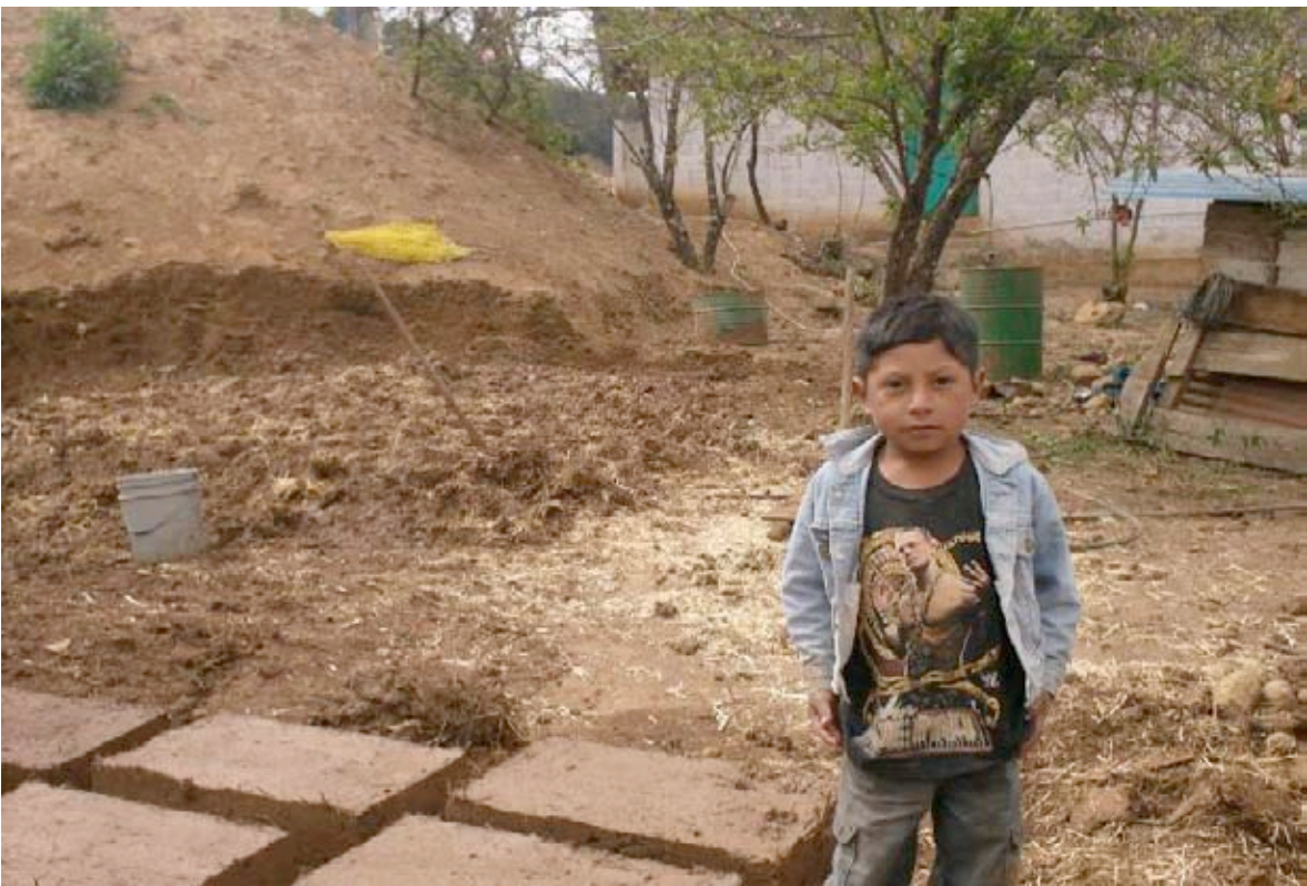
Photo No. 4: Barro (background) gathered for making adobe bricks.
