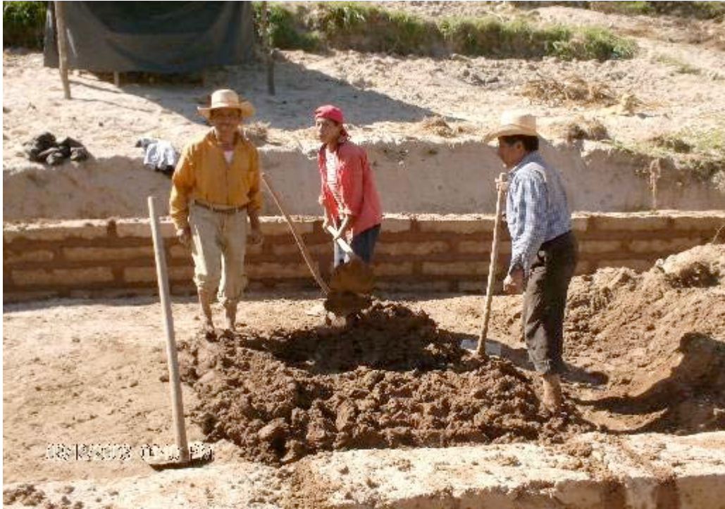
Photo No. 12: Preparation of adobe mortar.
