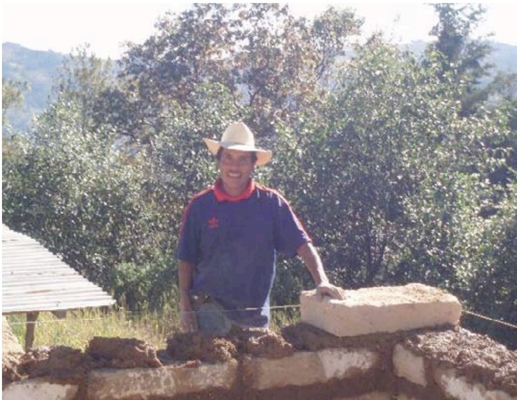
Photo No.13: Laying the adobe bricks with adobe mortar.
