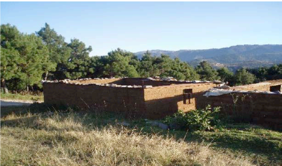
Photo No. 18 and 19: Drying of walls.
