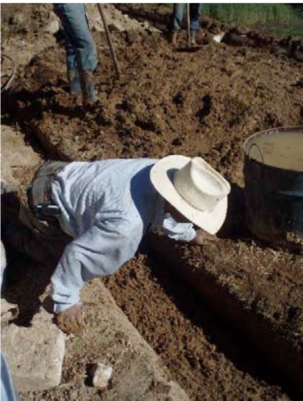
Photos No. 10 and 11: Placement of material to form the foundation.
