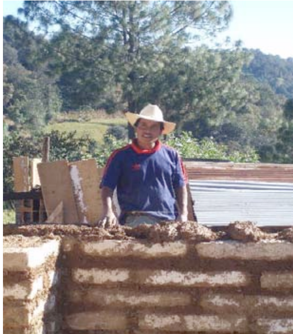
Photo No. 16: Horizontal string line that guides brick laying.
