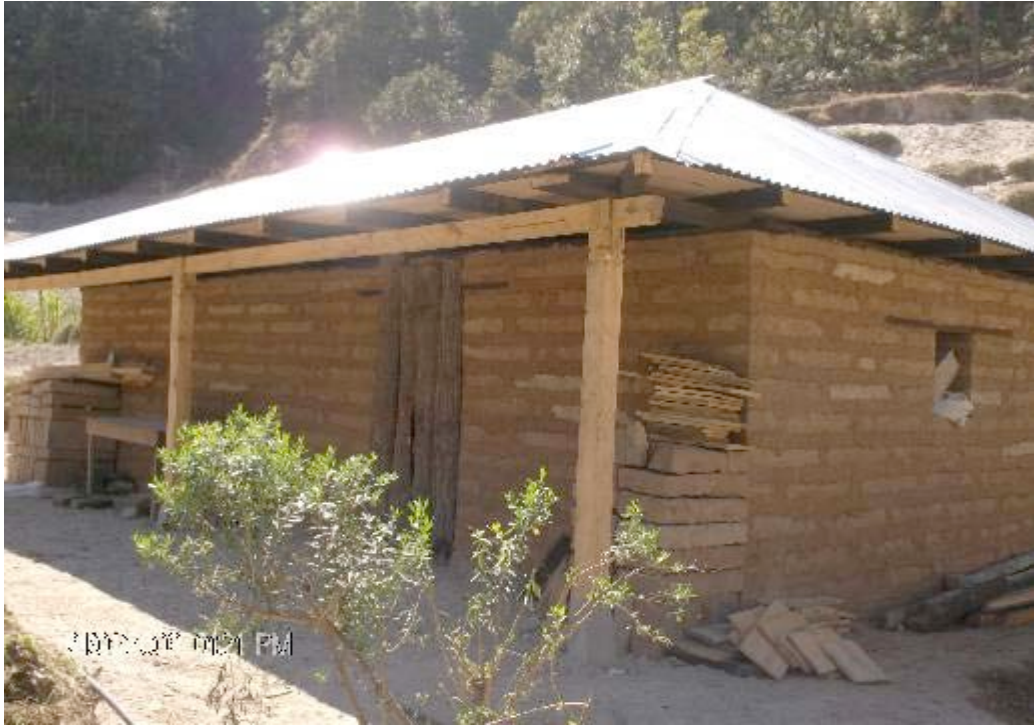
Photo No. 20: House with roof of corrugated metal sheets.
