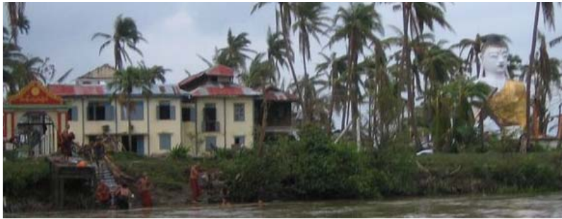
Monastery building still standing (intact). Pagodas and large Buddha Statues could be found nearby the building.
